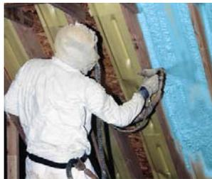
STYROFOAM™ Brand SPF Insulation meets IBC/IRC requirements for foam plastic insulation and is UL Classified Class I at 4 inches (UL 723). Also see ASTM C1029 and ASTM E84.
